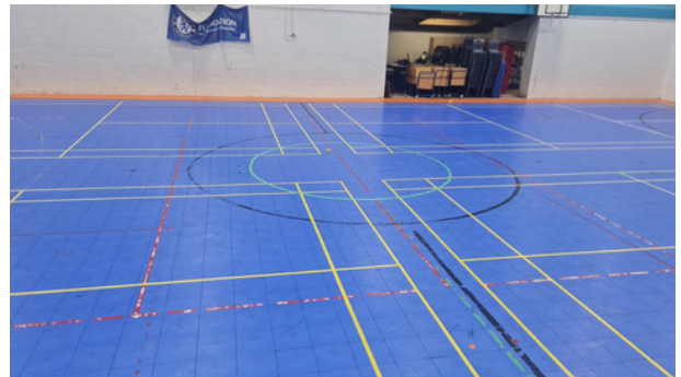
The hall mid renovation
